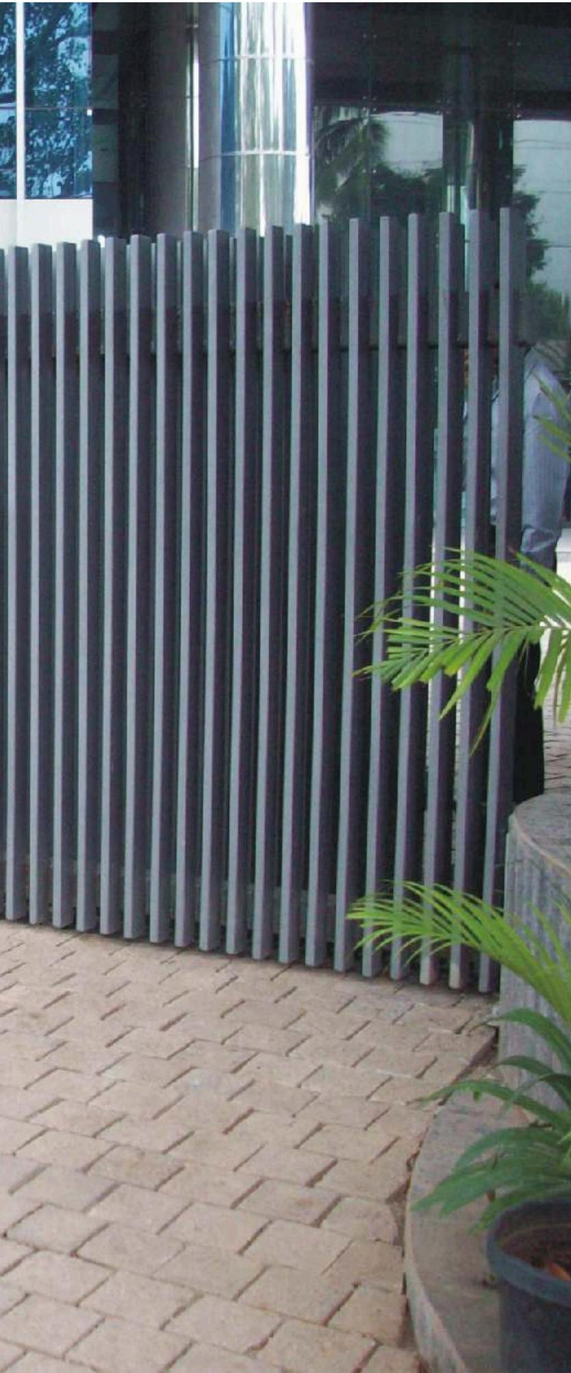
Gandhi gates are designed and fabricated with special square or rectangular hollow sections, along with MS sheets and flats assembled by high quality welding.
